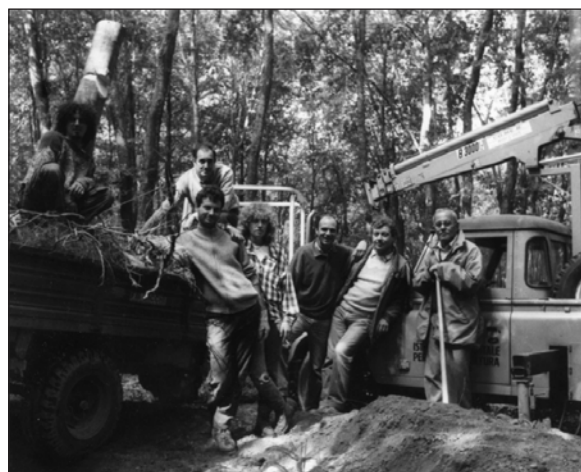
1988, the digging trial.
